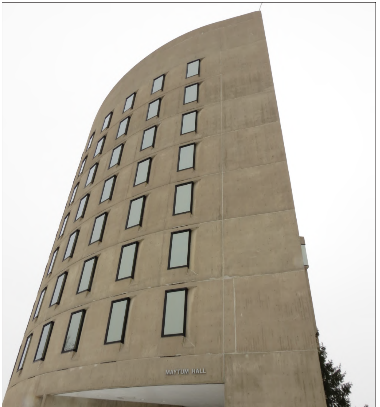
THOMAS WARMBRODT/ SPECIAL TO THE LEADER A SIDE-VIEW OF THE EXTERIOR OF MAYTUM HALL FOLLOWING ITS REOPENING TO THE PUBLIC.
