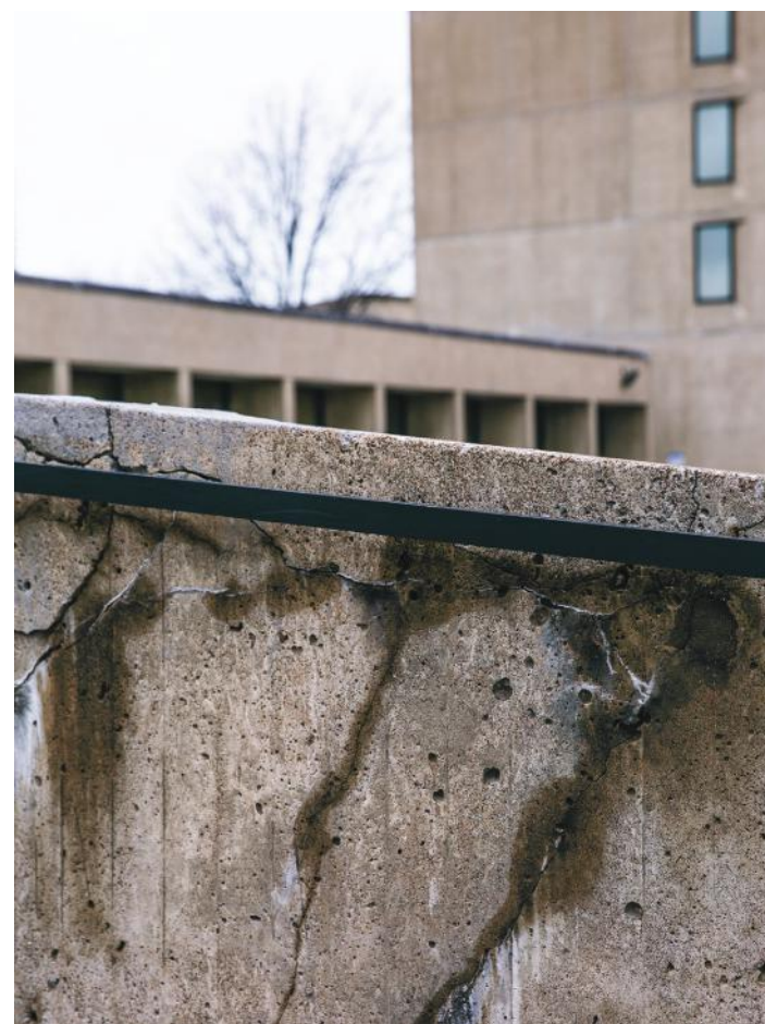
Deteriorating concrete on the stairs of Reed Library. Corey Maher/Photo Editor
