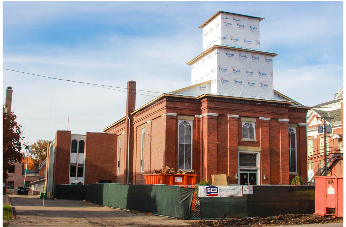
Progress is being made on the reconstruction of the church.
