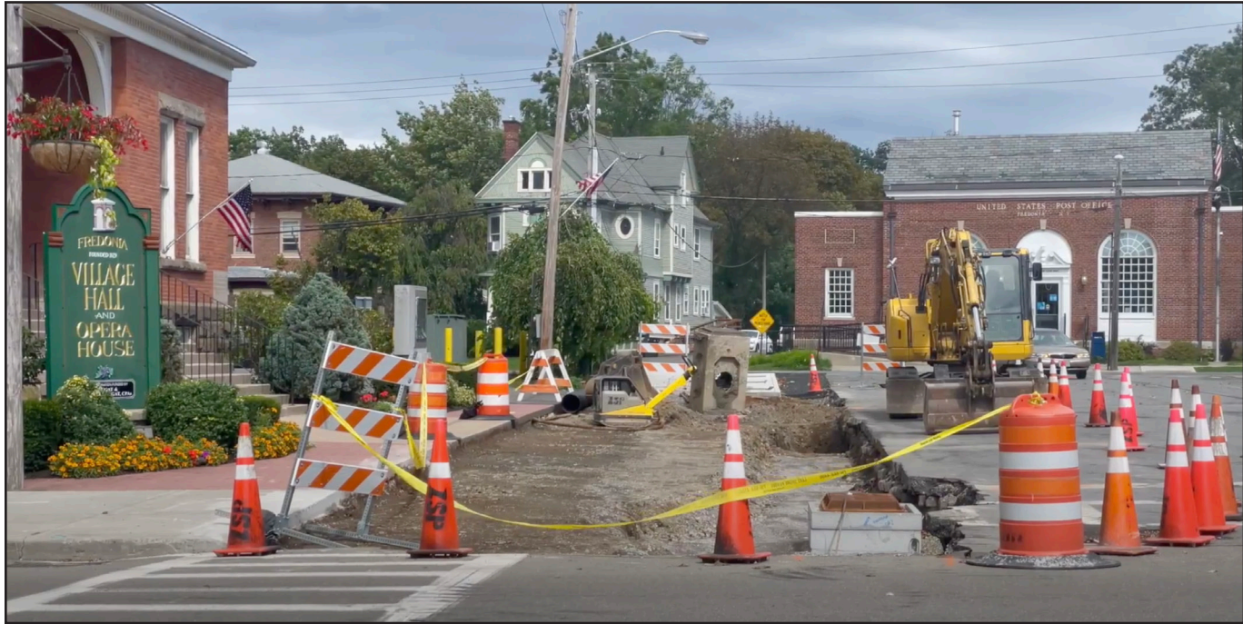
Construction on Church Street. Photograph by Analise Healy.
