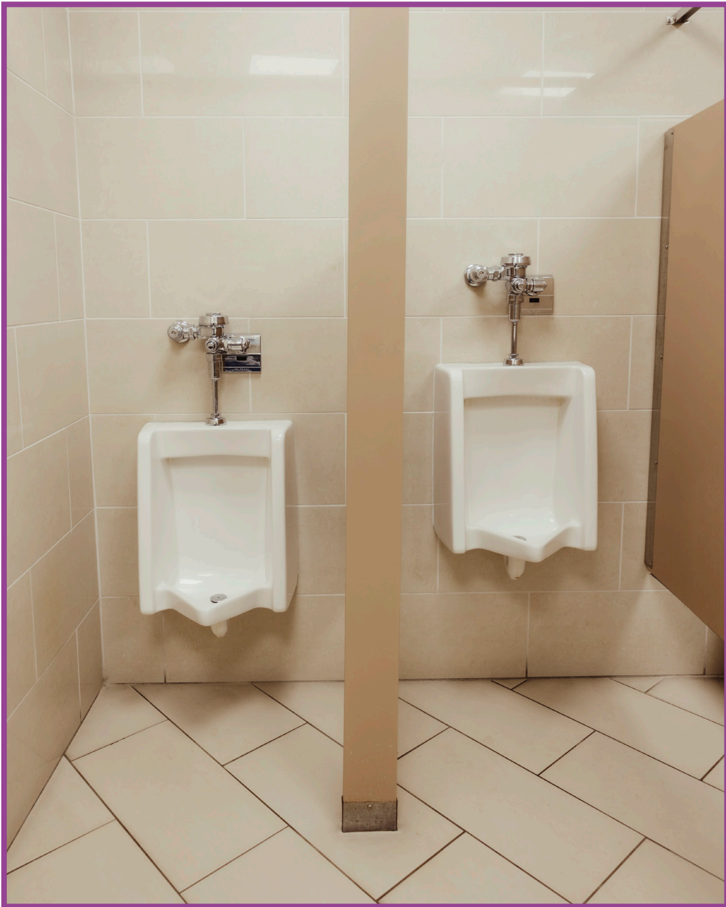
Williams Center Bathroom. Photograph by Derek Raymond.
