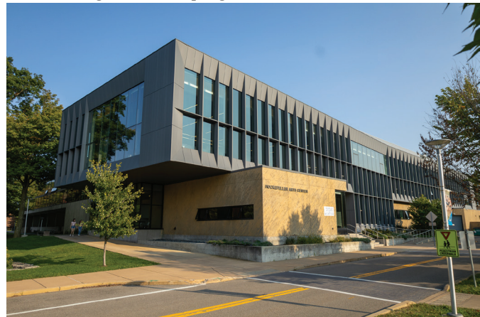
Rockefeller Arts Center, one of the buildings where classes of the discontinued majors take place.
