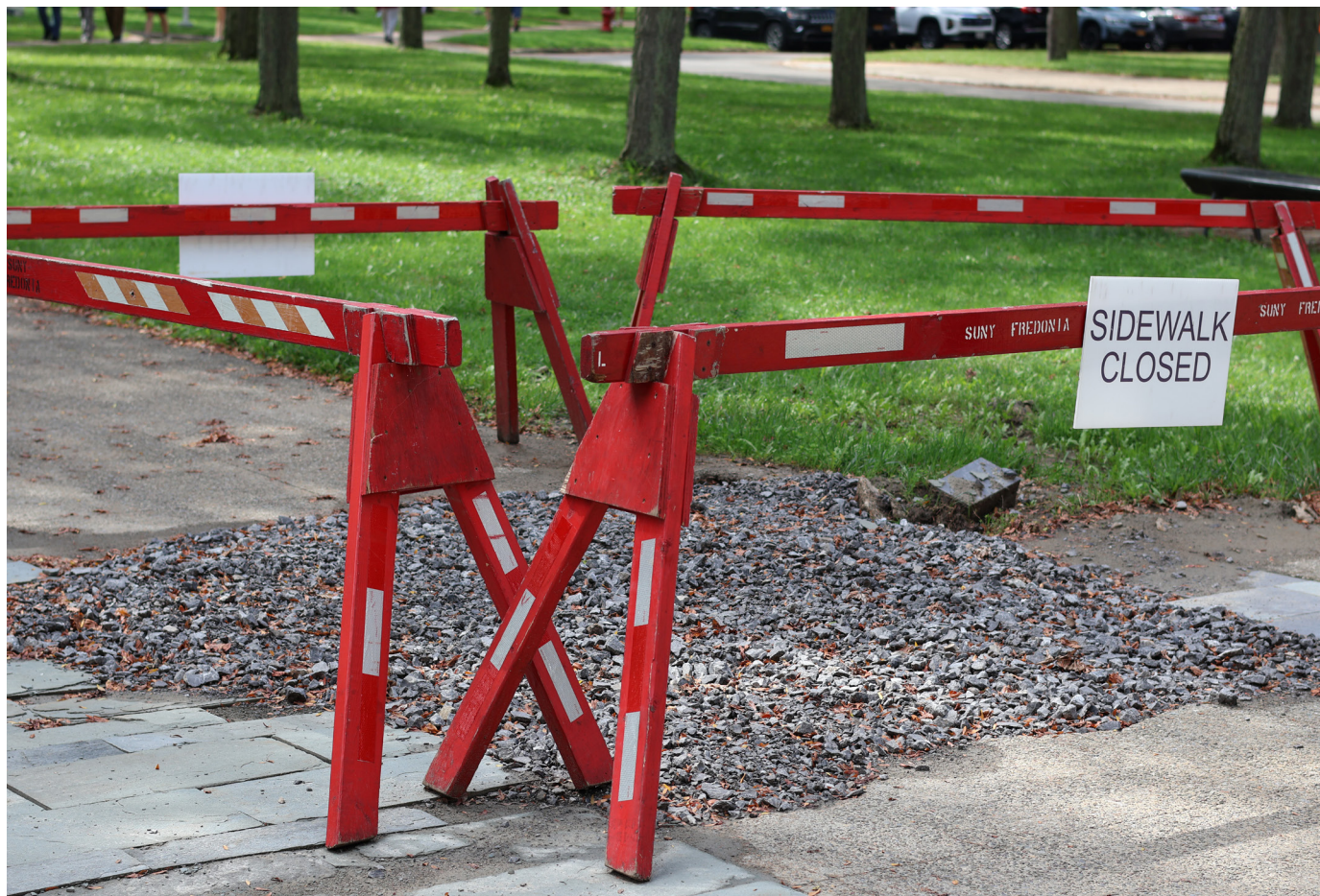
Sidewalk blocked off in front of McEwen Hall. Photo by MARS ARENSEN | Special to The Leader
